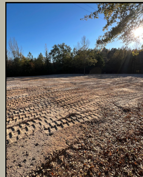
Land Grading for a new parking area
