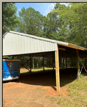
Expanded Pole Barn for Events
