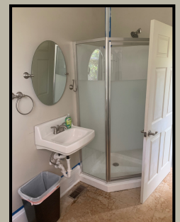
New Bathrooms with Showers
