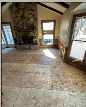
Farm House Renovations
