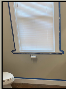
New Windows, Paint, and Sewage System
